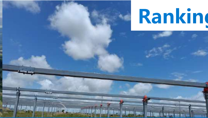
High Temperature and Humidity Cambodia — 78 MW
