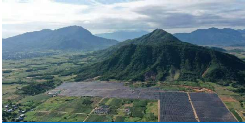
10% Slope Terrain Vietnam — 35 MW
